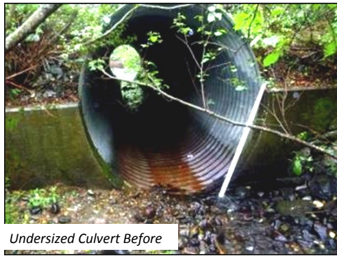
Rusted Culvert Bottom
