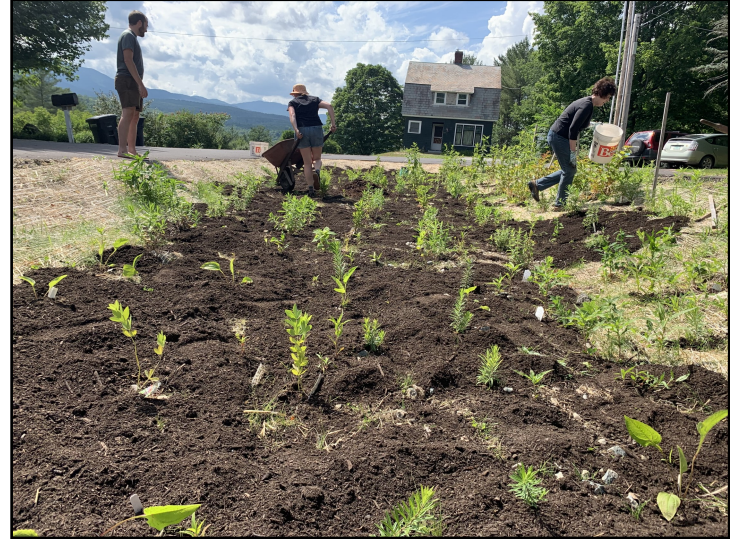
Bioretention Raingarden in Hyde Park
