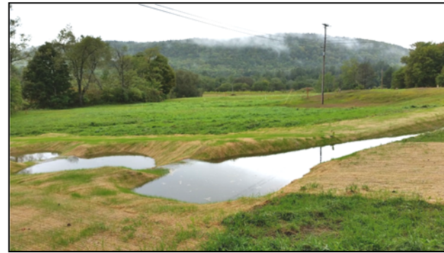
Step Pool Conveyance System off Morey Road
